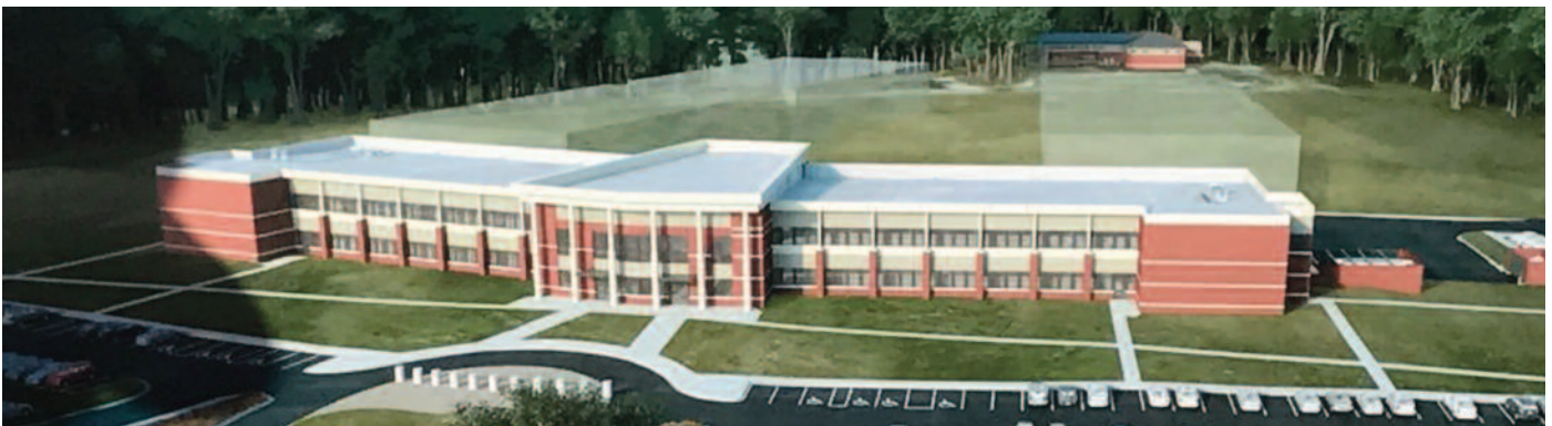
AFRC Consolidated Mission Complex project that wrapped up in Robins AFB, Georgia last year.
