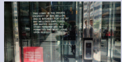
101 Barclay is one of the sites violating existing regulations on POPS (NYC Comptroller Office)
